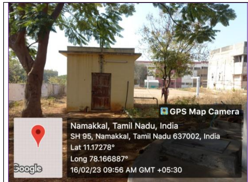
Bore wells water room
